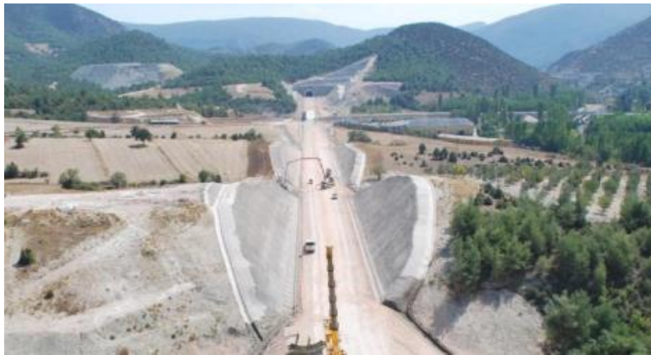
Fig. 4. Perspective of a double track railway route through a cut (UDH, 2012).
