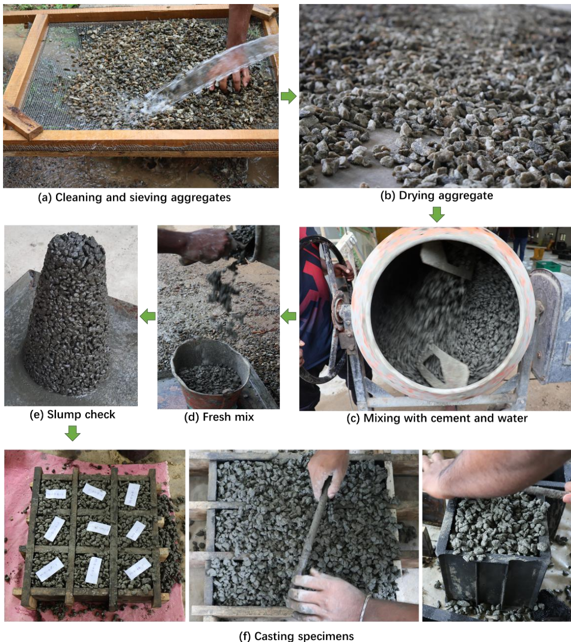
Fig. 2. Casting procedure of pervious concrete mix.
