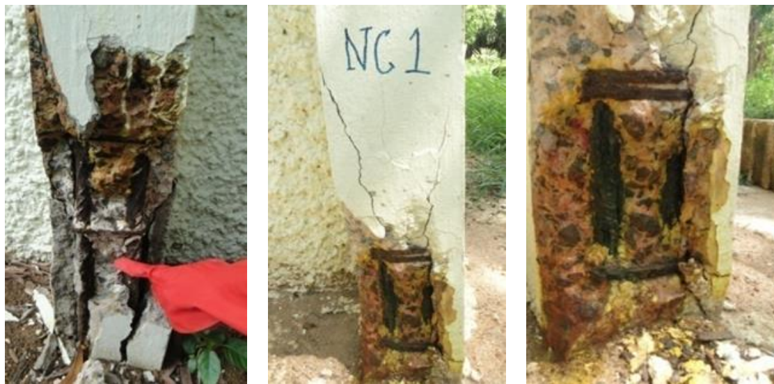
Fig. 6. Colorimetric method to check free and bound chloride on the exposed structural member.
