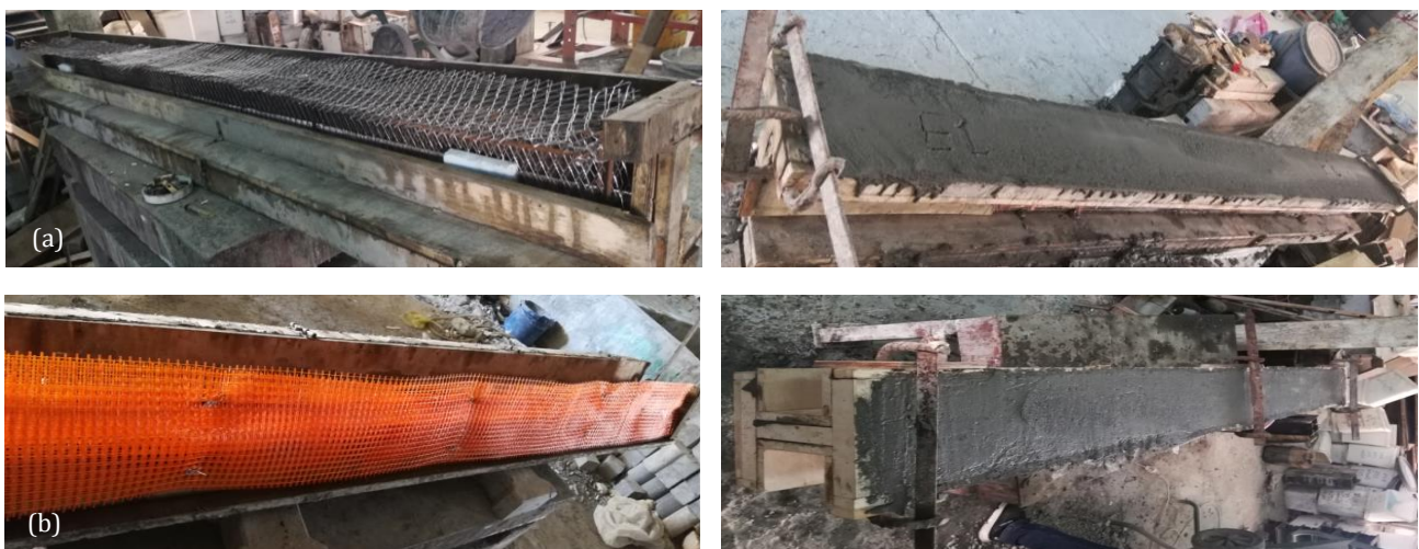
Fig. 3. The configuration of meshes employed in the preparation process: (a) Beams featuring expanded metal mesh reinforcement; (b) Beams reinforced with Gavazzi mesh.
