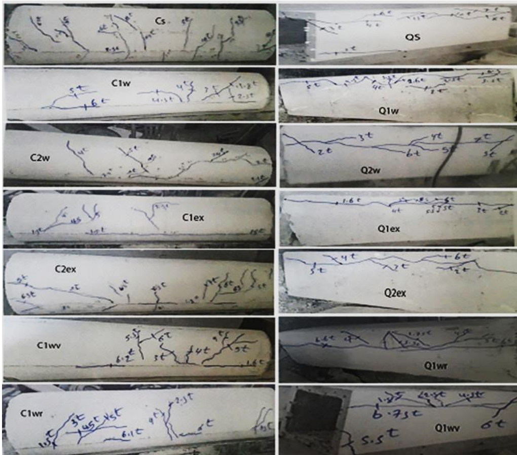
Fig. 13. Cracking pattern of tested beams.
