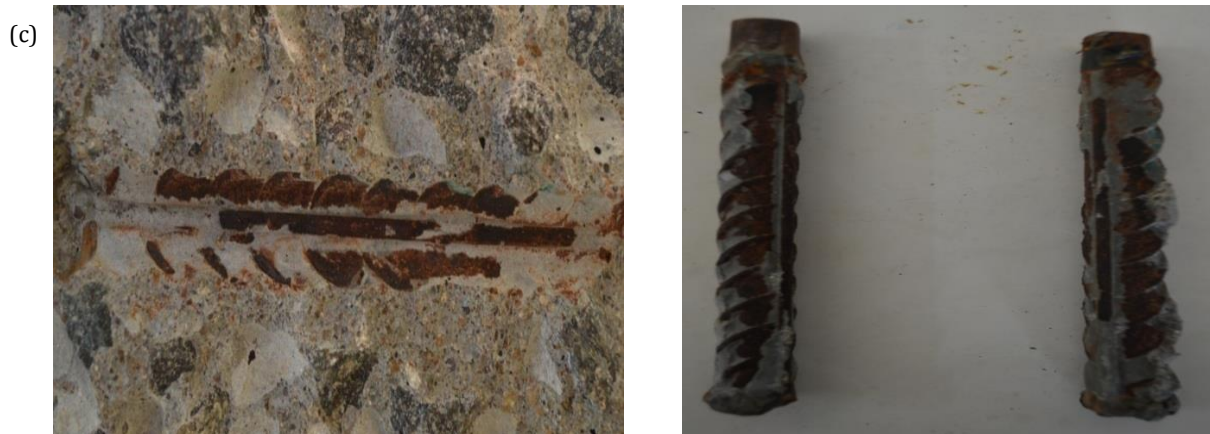
Fig. 14. (a) Comparison of cracking time for nano-modified CPAC coated (single and double) and uncoated rebar in control concrete; (b) Cracked specimens (uncoated, single and double coated) after subjected to accelerated corrosion test; (c) Condition of concrete and coated rebar at the end of accelerated corrosion test.
