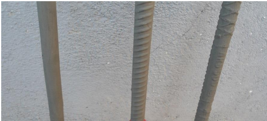
Fig. 4. View of nano-modified cement polymer anticorrosive coated rebars.
