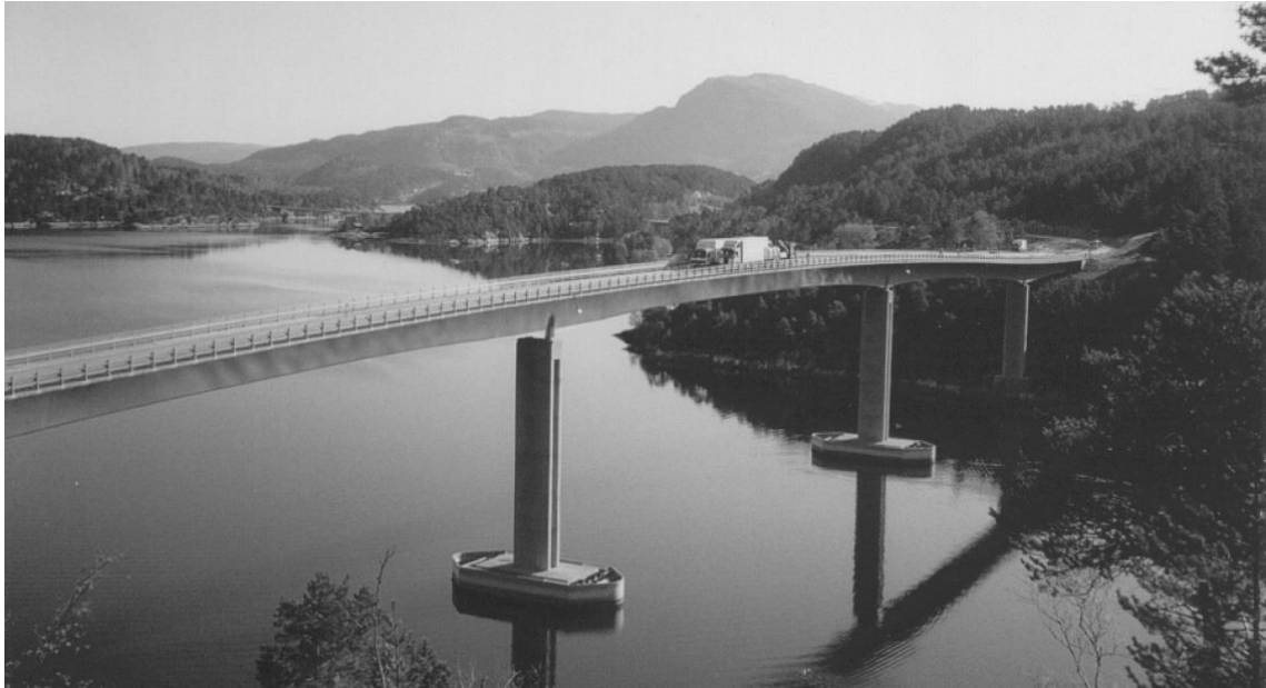
Fig. 12. Mjosundet Bridge used for the field trials.
