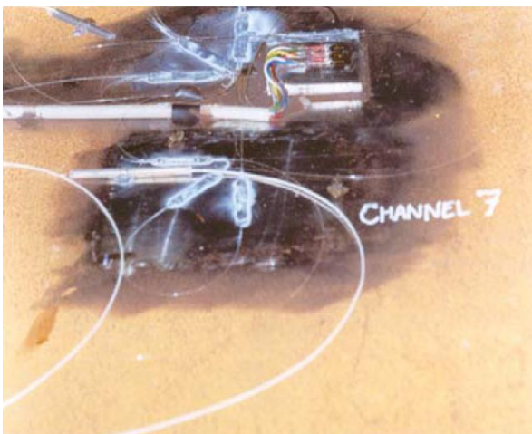
Fig. 2. Installed optical fibre sensors on steel structure.
