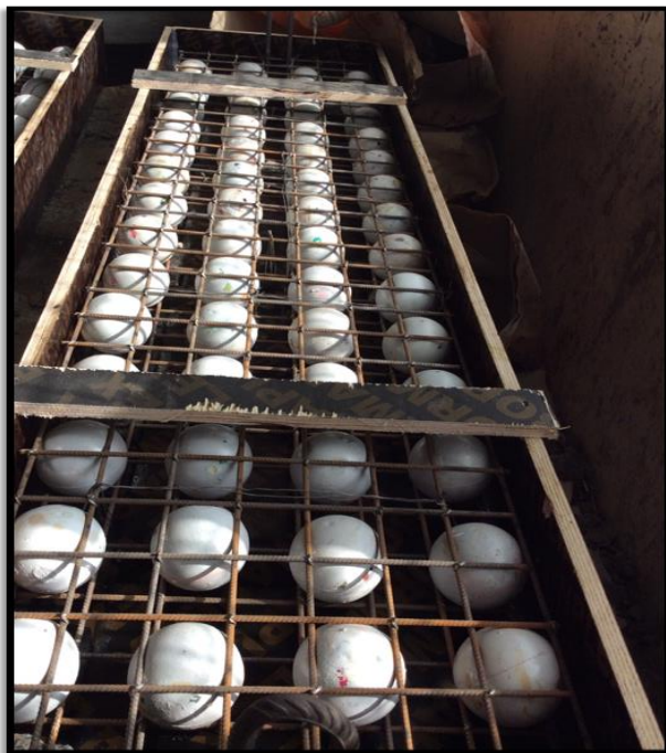
Fig. 1. Preparation of bubbled slab.
