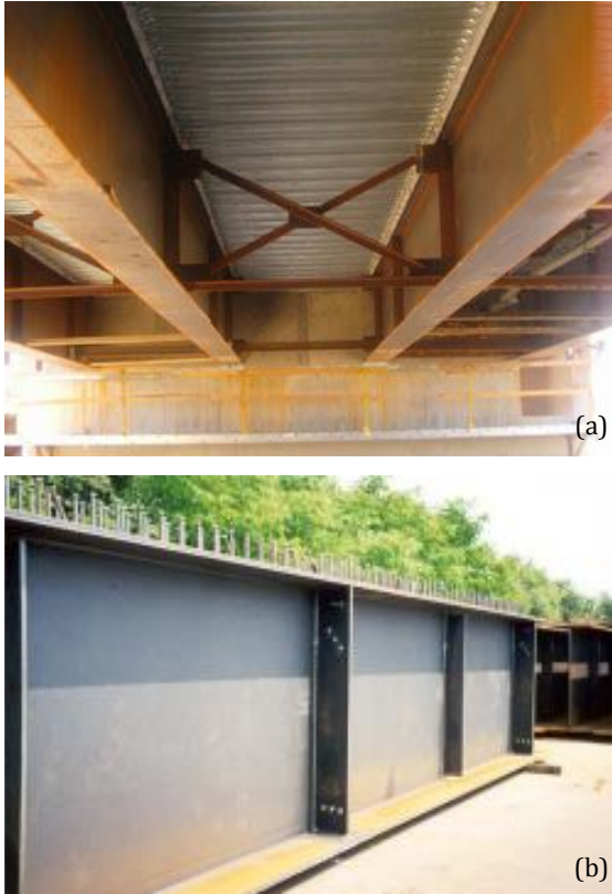
Fig. 1. (a) Typical steel-concrete composite bridge, (b) Steel girder with stud shear connectors.
