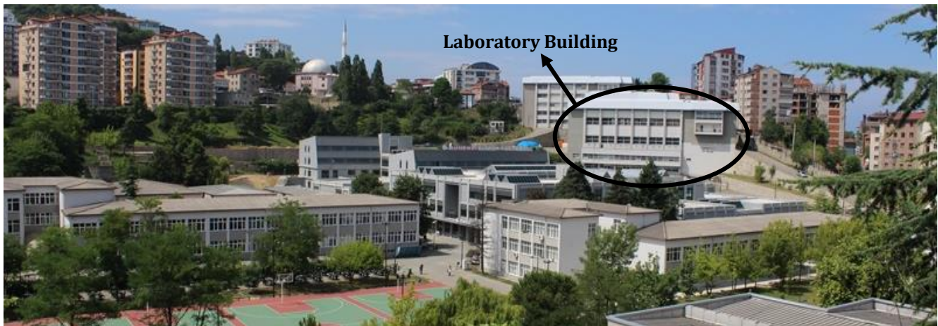
Fig. 1. View of the Laboratory Building.
