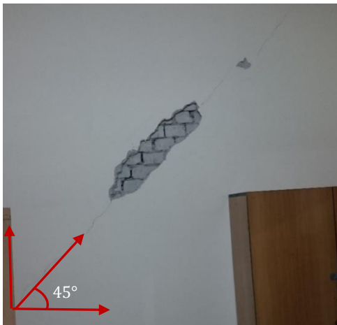
Fig. 11. Shear cracks on load bearing walls in the ground floor of the Block B.
