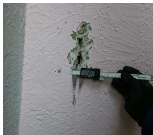
Fig. 8. Expansion joint between two buildings (11.55 mm < 30.00 mm).
