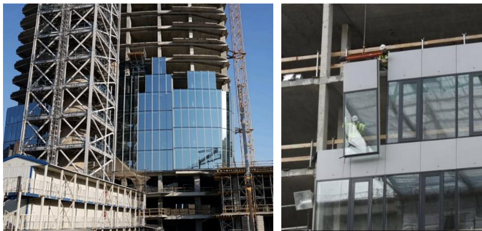
Fig. 2. Unitized curtain wall system (UCWS) (Web-2 2022).
