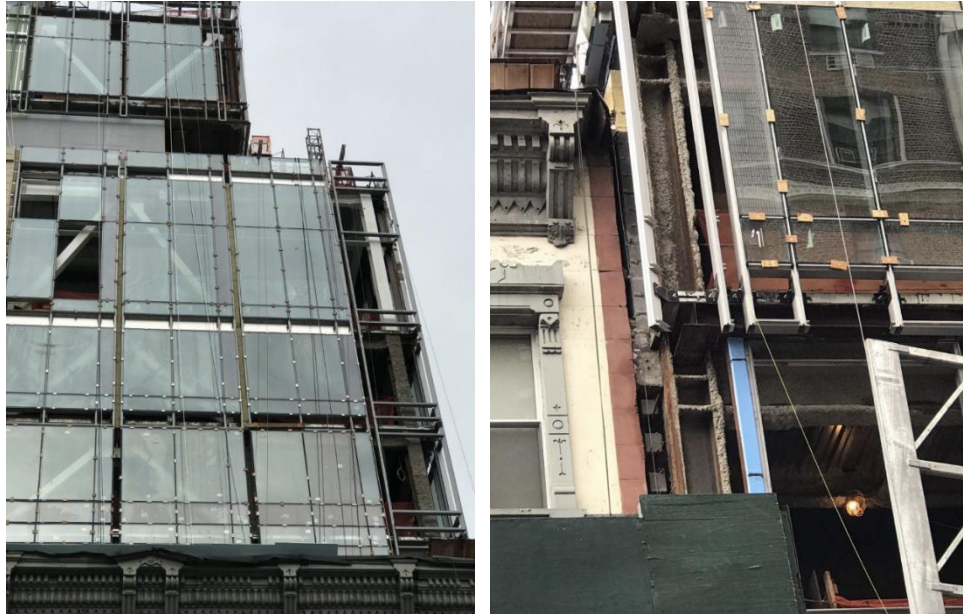
Fig. 1. Stick curtain wall system (SCWS) (Web-1, 2022).
