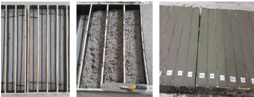
Fig. 2. Appearance of the concrete bollards while casting and concrete working.
