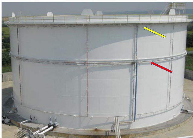
Fig. 2. A cylindrical steel tank with a PSR and a single SSR (courtesy of Dr. Zdravkov).
