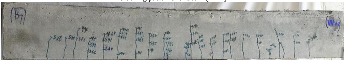
Cracking patterns for beam (WV2)
