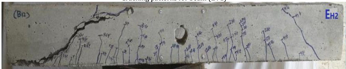
Cracking patterns for beam (EH2)
