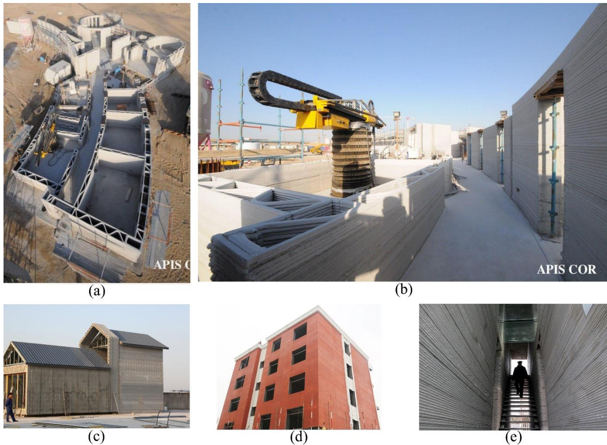
Fig. 1. Examples of large-scale 3D-printed concrete construction: (a),(b) Dubai “Office of the Future” printed by Apis Cor (Archdaily 2019); (c) Single-story houses by WinSun (Architectsjournal 2014); (d) WinSun’s five-story apartment building (Winsun3d 2015); (e) Interior corridor of a 3D-printed villa (Zoey 2018).
