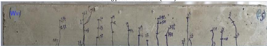
Cracking patterns for beam (WV1)
