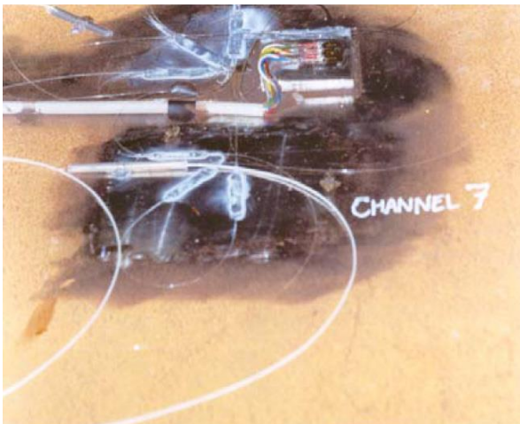
Fig. 2. Installed optical fibre sensors on steel structure.
