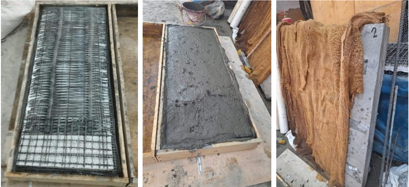
Fig. 12. Preparation, casting, and curing of the tested plates.
