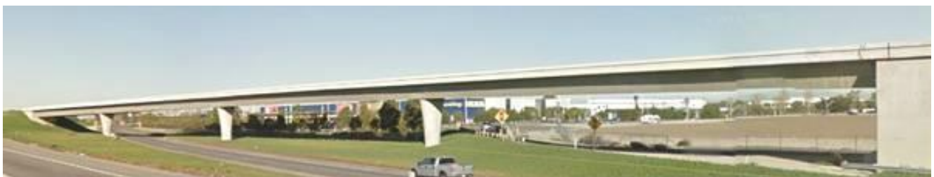
Fig. 1. A view of the Fairview Road On-Ramp Overcrossing (FRO) Bridge.
