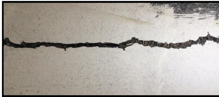
Fig. 8. Ultimate failure crack.
