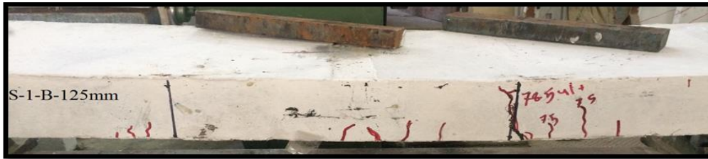
(a) Flexural failure of (S-1-B-125mm)
