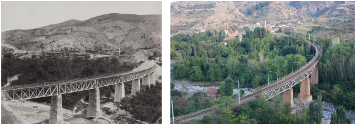
Fig. 1. General views of the Bekdemir railway bridge.
