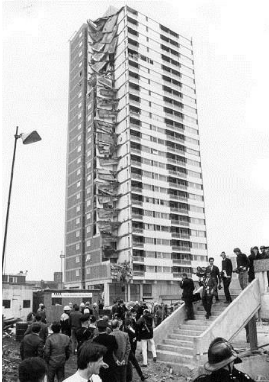
Fig. 1. Ronan Point apartment building after collapse (Pearson and Delatte, 2003).
