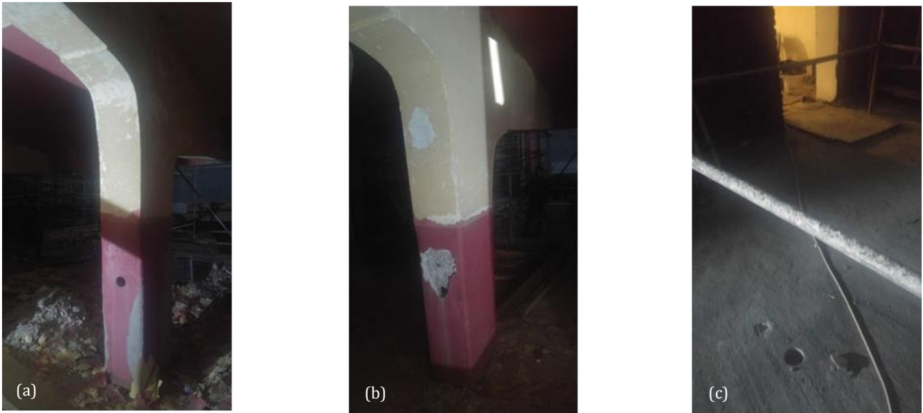
Fig. 4. Core samples taken from the structure: (a) Main column S41; (b) Main column S42; (c) Balcony flooring.
