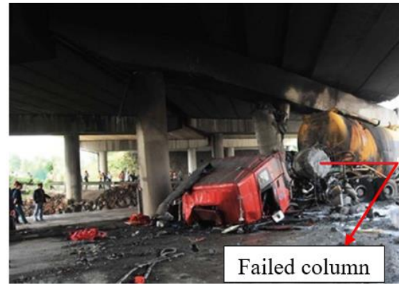
Fig. 1. Collapse of structure/structural member due to impact load (Do et al. 2018).
