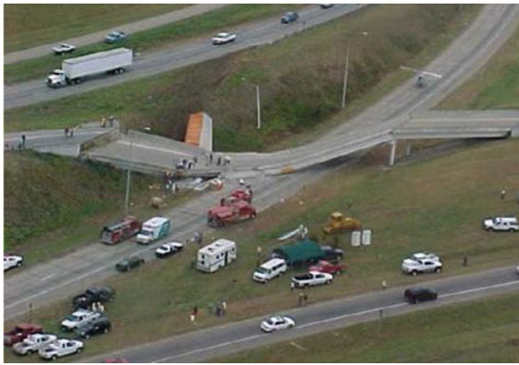
Fig. 1. Collapse of structure/structural member due to impact load (Do et al. 2018).
